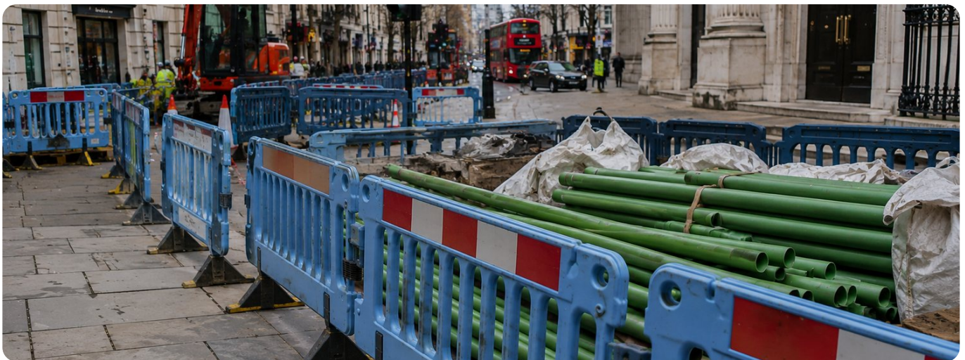
The build that ran on cheap money: fibre ducting laid through a city street. When rates rose, the digging that reshaped Britain's pavements became the debt that is now reshaping its ownership. Image: BroadbandSwitch.uk.
